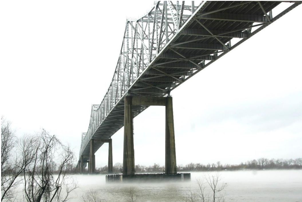
Character-defining Feature Photo 2: Caisson-constructed piers.
