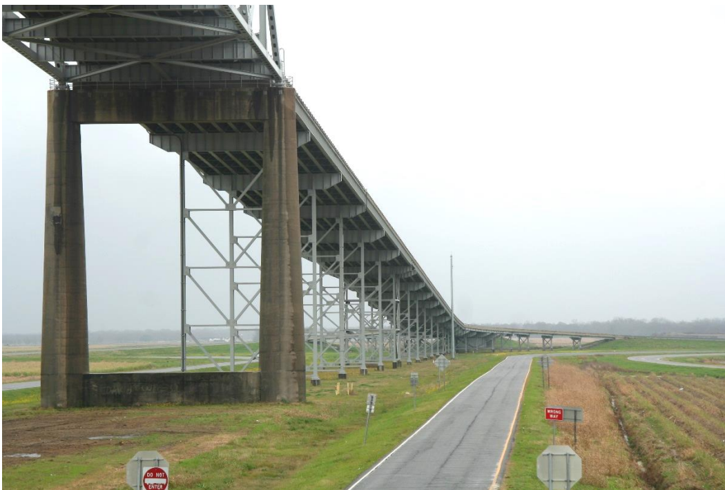
Condition Photo 12: Pier 7 and easterly approach spans.
