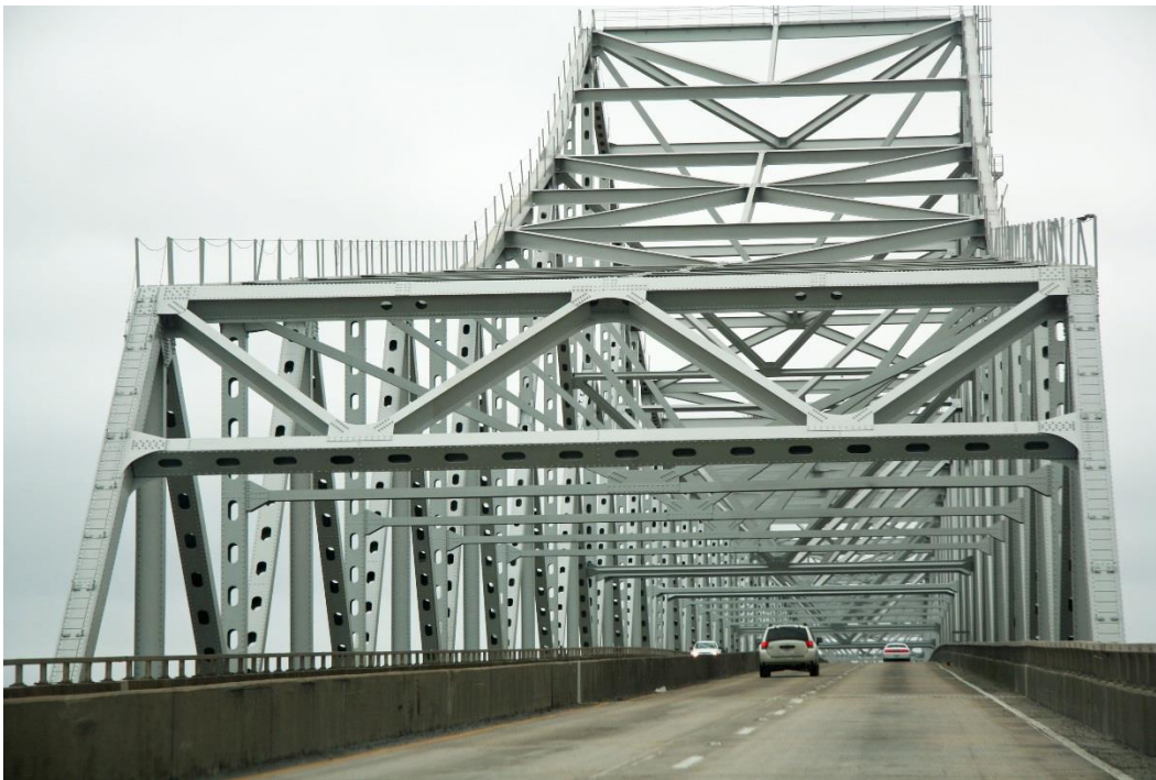
Condition Photo 10: Eastbound roadway through truss spans.
