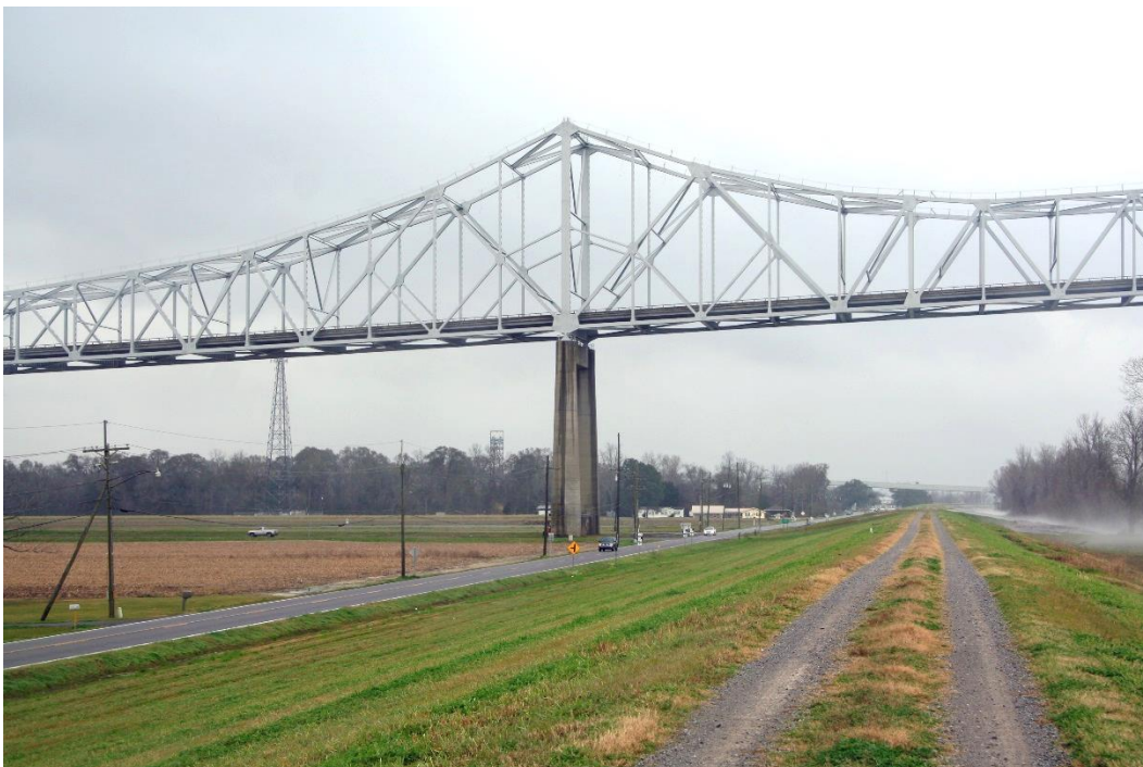
Condition Photo 16: Pier 6 and truss span over LA 44 and east levee.
