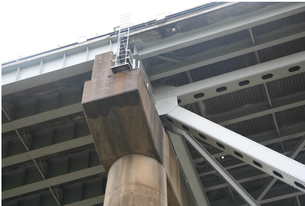
Condition Photo 2: Approach span 17 and deck truss span 18 at Pier 1.
