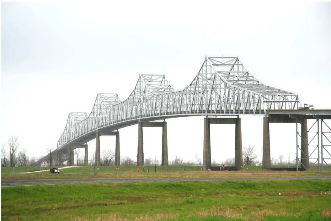
Character-defining feature Photo 1: Design and construction of a continuous Warren through truss. The Warren truss features diagonal members to withstand both tensile and compressive forces, and added verticals for bracing.
