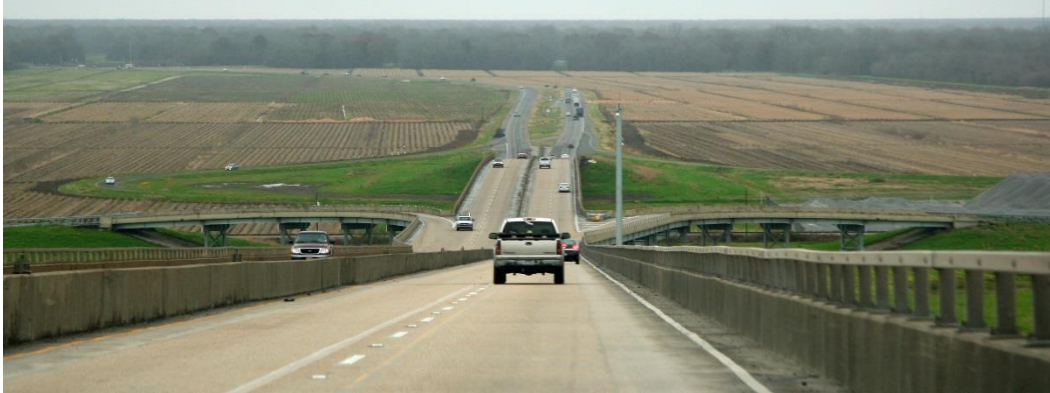
Condition Photo 11: Eastbound roadway looking east at easterly Y-split in ramps at end of bridge.
