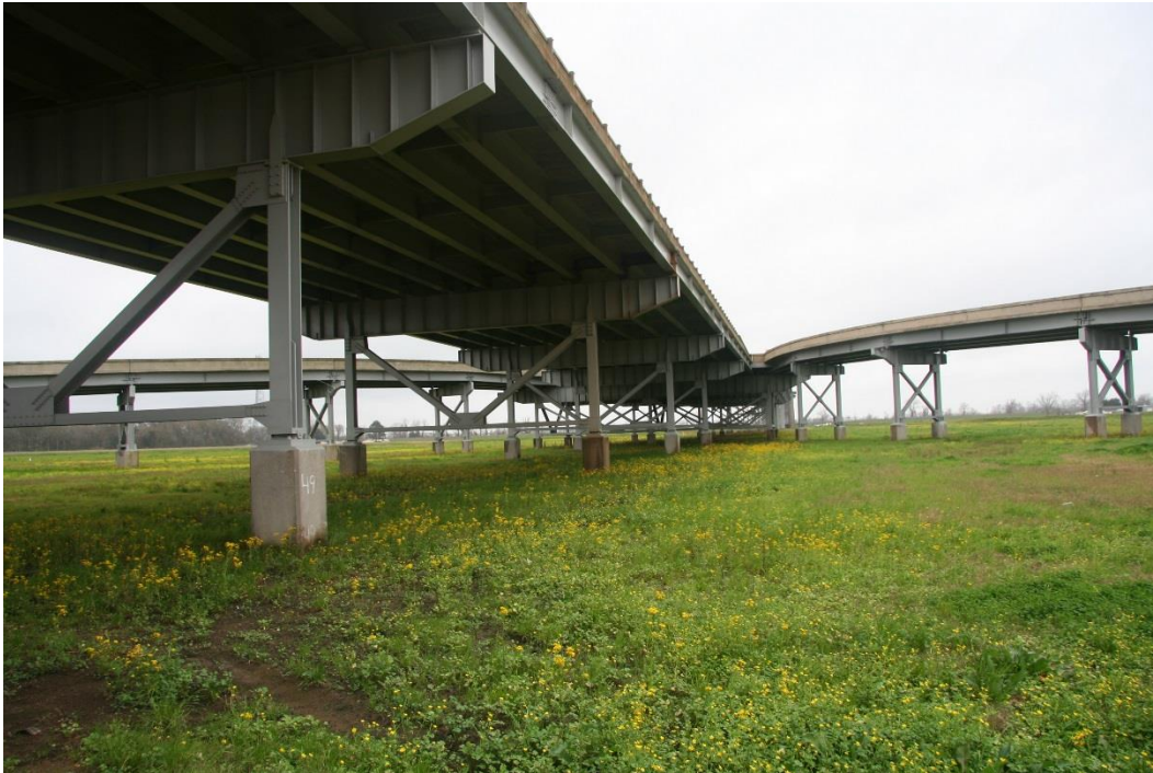
Condition Photo 15: Y-shaped split of ramps at east end of bridge.
