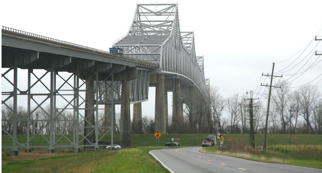
Condition Photo 5: Westerly approach spans and truss span over LA 18.
