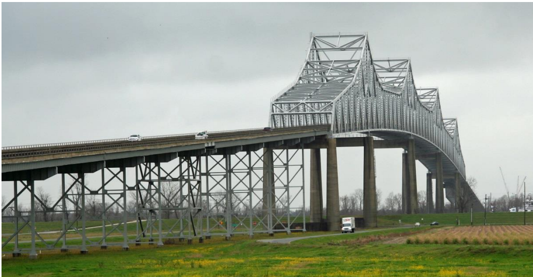
Condition Photo 18: Overall view of bridge looking west.
