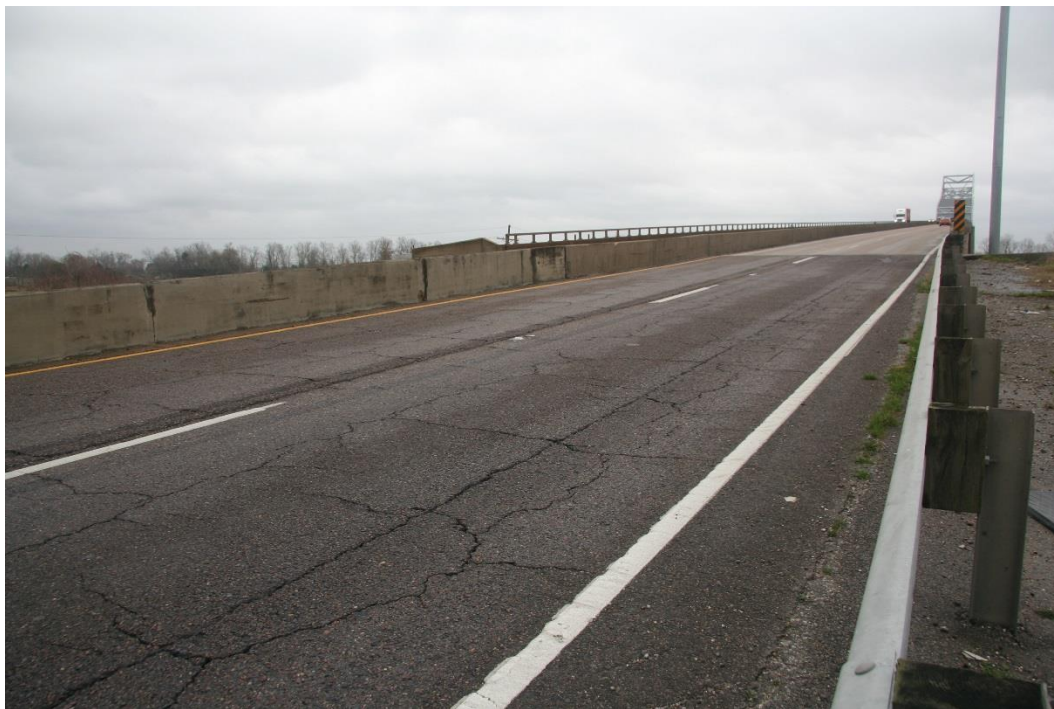
Condition Photo 6: Eastbound approach roadway at west end of bridge.
