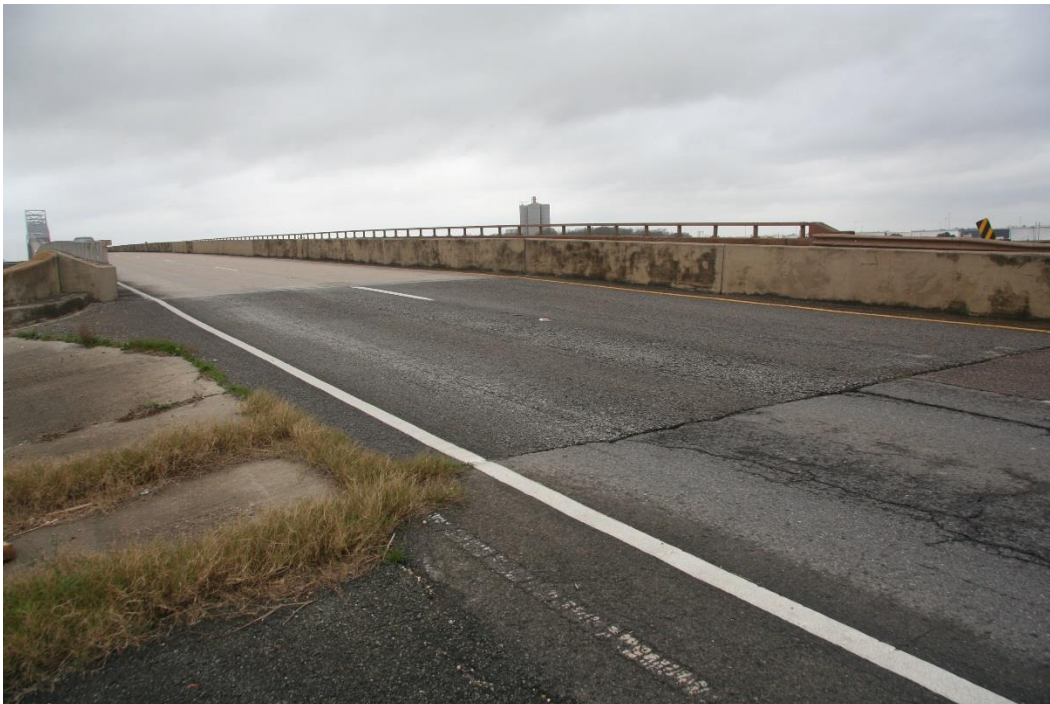
Condition Photo 20: Approach roadway at east end of eastbound roadway.
