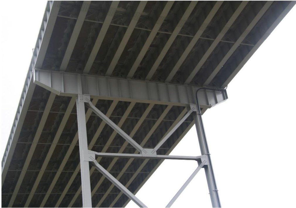
Condition Photo 1: Westerly approach spans at Bent 22.
