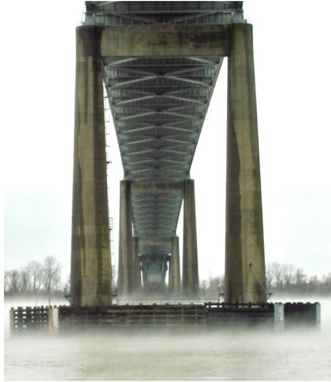
Condition Photo 13: Fender protection system at Pier 5.
