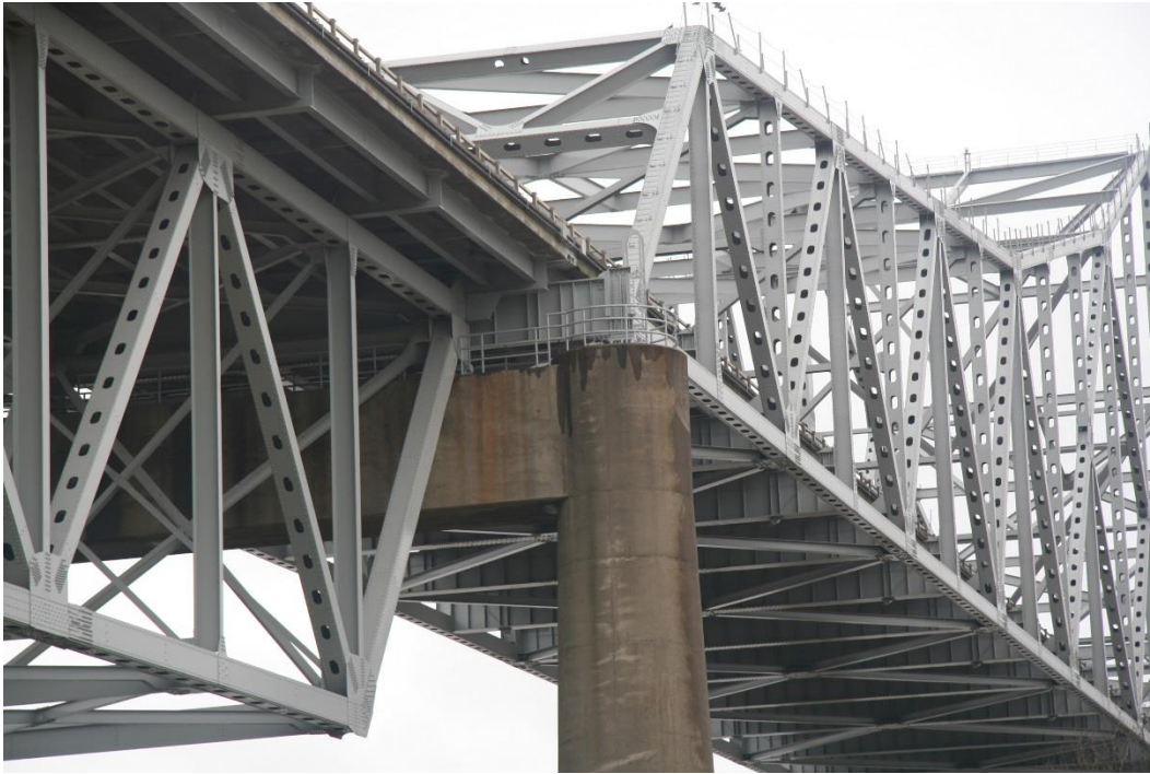
Condition Photo 3: Deck truss span 18 and main truss span 19 at Pier 2.
