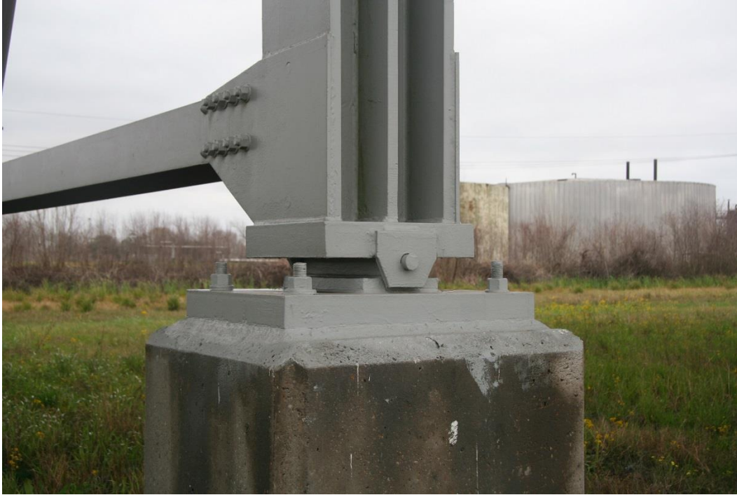
Condition Photo 7: Column base detail for westerly approach spans.
